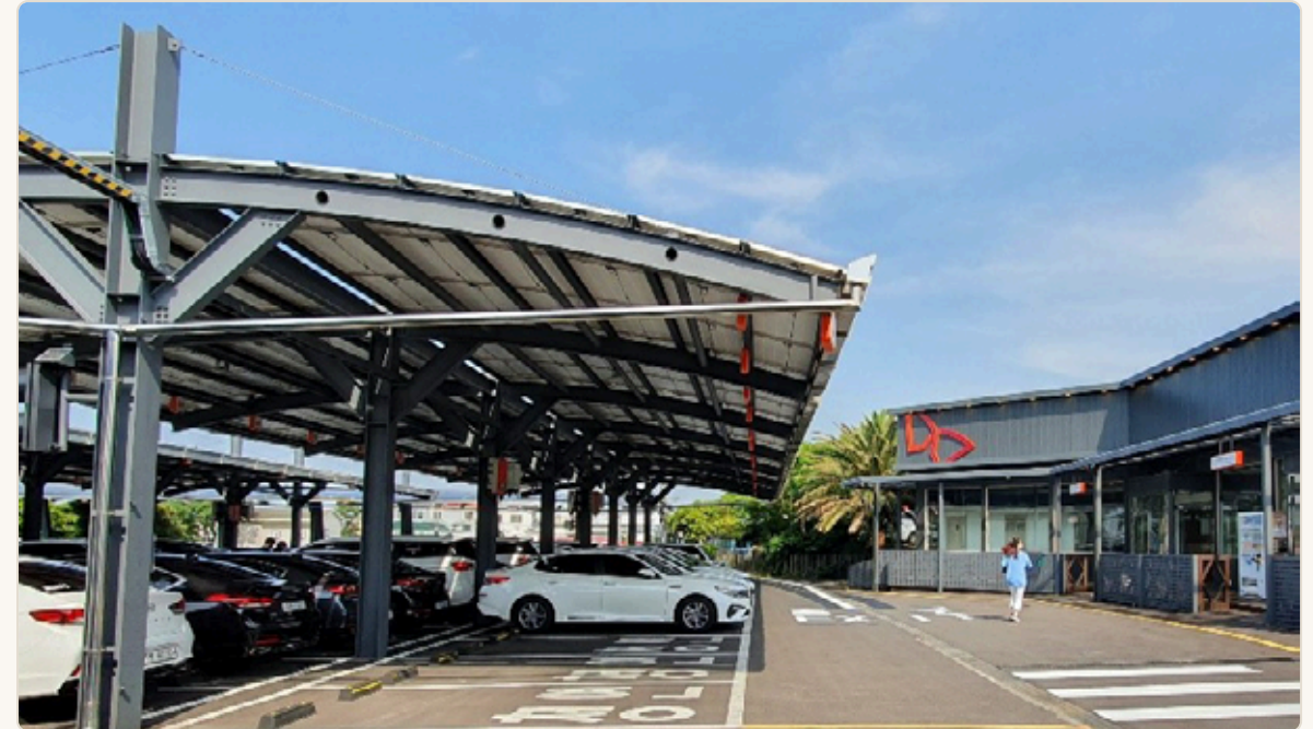
Solar-panel canopy over the Jeju branch parking area.
